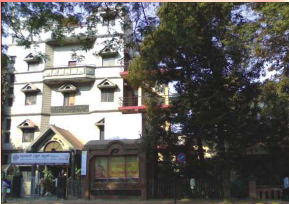
“ The exquisite 98-year old lady of Chamarajpet ! ” ----- The headquarters of the erstwhile Bangalore Central Co-operative Bank Ltd., now taken over by SVC as its Chamarajpet Branch.
